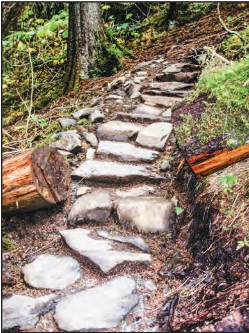
Trail Class 3: Constructed Features —Constructed features such as walls, steps drainage, and raised trail, may be common and substantial.
